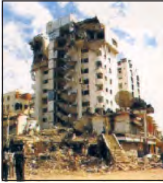
Fig. 3.3a: Destruction caused by an Earthquake in Gujarat
